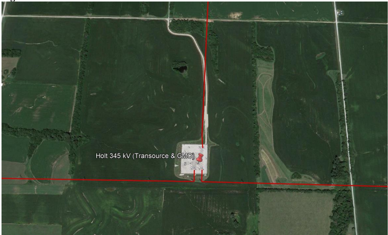
Figure 29 – Holt 345kV Substation
