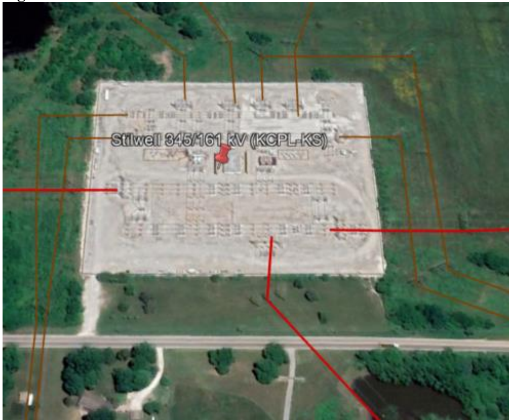
Figure 28 – Stilwell 345 kV substation
